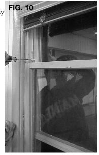
Cut foam sash seal to window width and place into space between upper and lower sashes to seal out air infiltration
