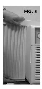
Keeping a firm grip on the air canditioner. carefully place unit into window opening so bottom of air conditioner frame is against window sill (FIG. 6). Carefully close window behind top rail on unit
